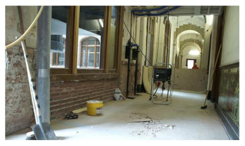
In this corridor we reconstructed the Art Nouveau tile designs from 1901 over a length of 20 meters. The tiles on the left side of the hallway were completely missing.
